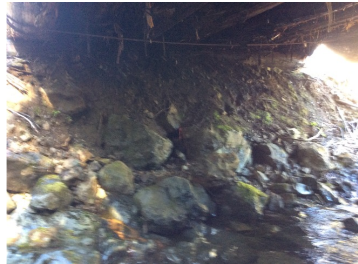
Left Bank Abutment when facing downstream
