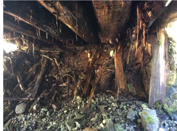
Right Bank Abutment when facing downstream
