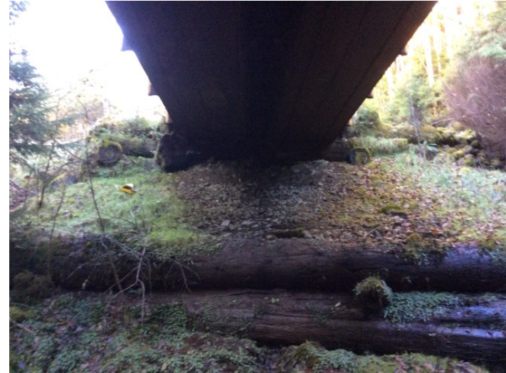
Right Bank Abutment when facing downstream
