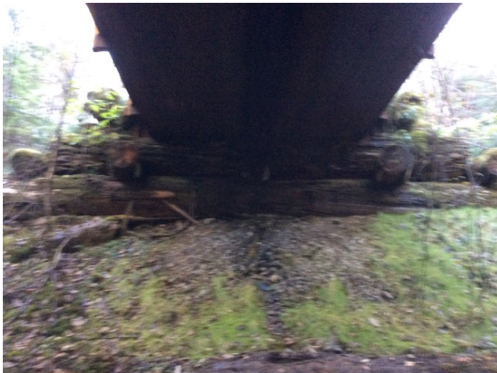
Left Bank Abutment when facing downstream
