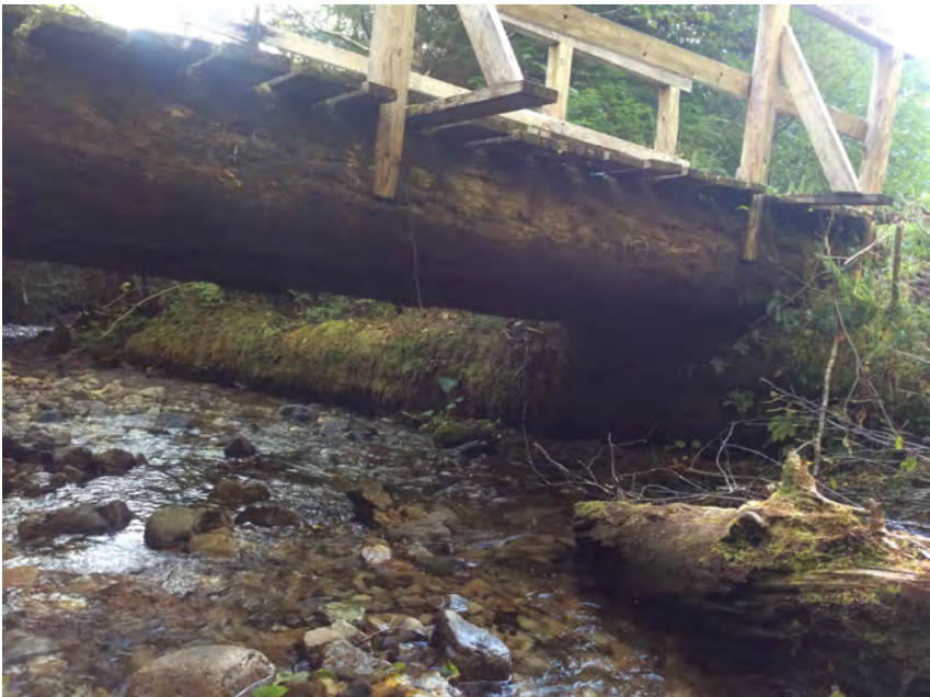
Right Bank Bridge 1 Abutment when facing downstream
