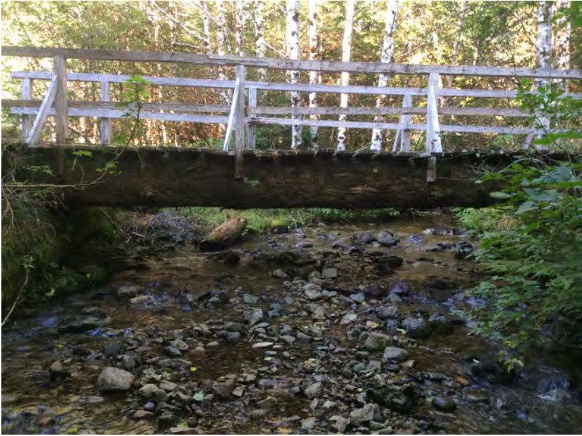
Bridge 1 Downstream Profile
