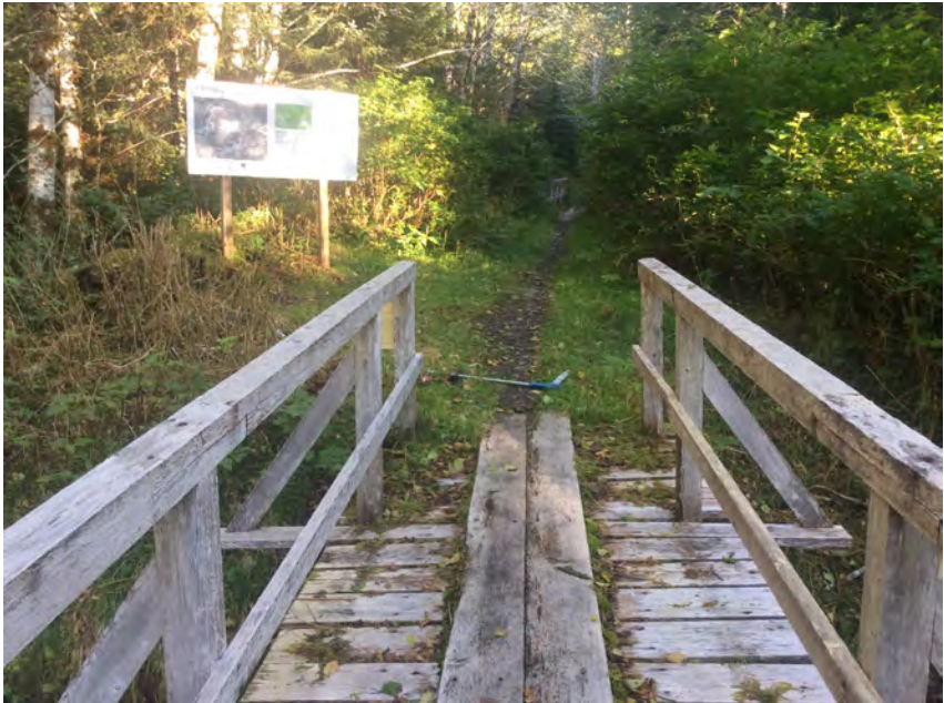
Centre of bridge 1 to river left approach
