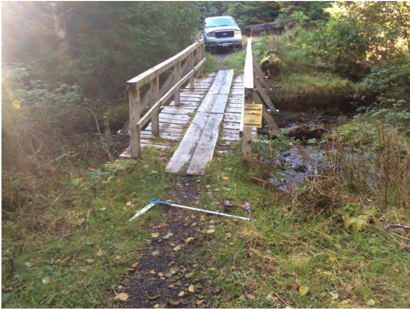
River right approach to Bridge 1
