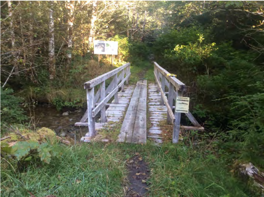
River right approach to Bridge 1
