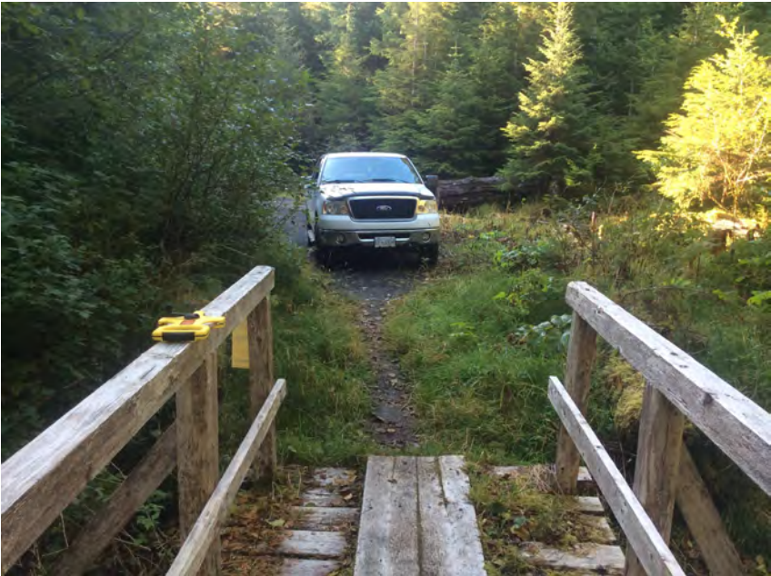
Centre of bridge 1 to river right approach
