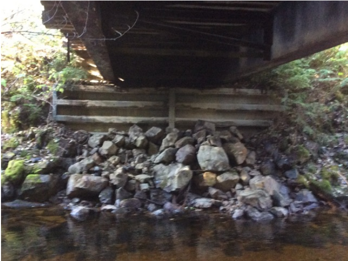
Right Bank Abutment when facing downstream
