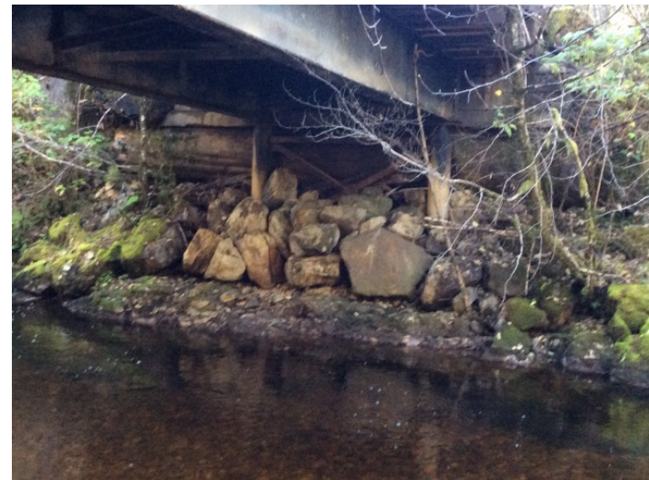
Left Bank Abutment when facing downstream
