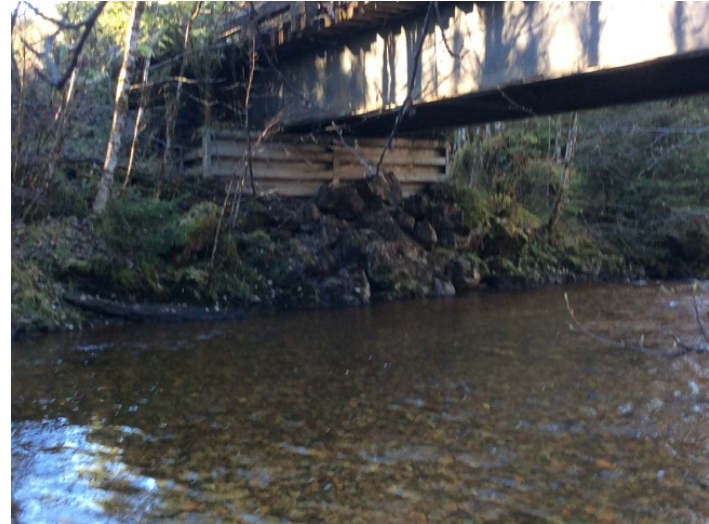
Left Bank Abutment when facing downstream
