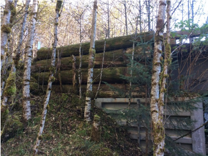
Right Bank Abutment when facing downstream
