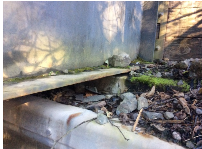
Right Bank Abutment when facing downstream
