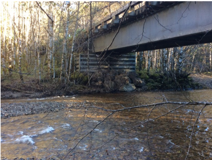
Right Bank Abutment when facing downstream
