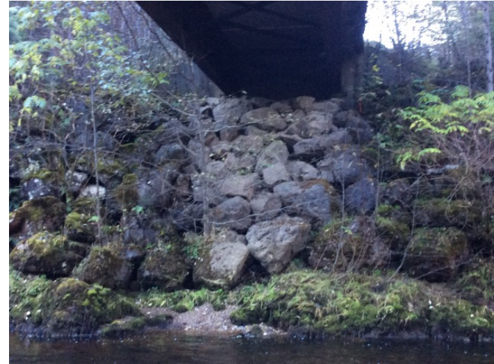
Left Bank Abutment when facing downstream
