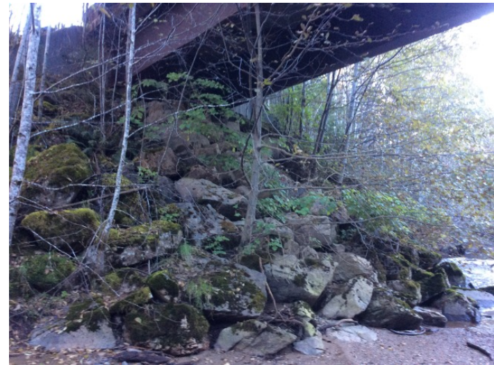
Right Bank Abutment when facing downstream
