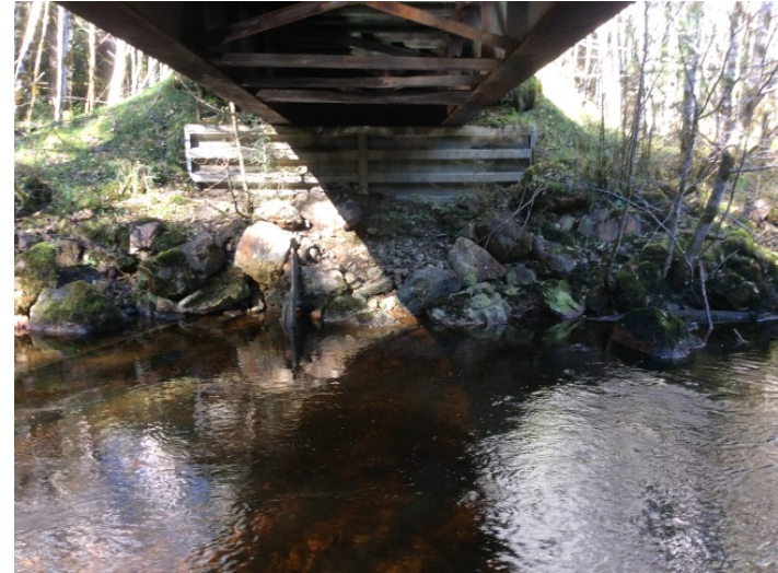
Right Bank Abutment when facing downstream
