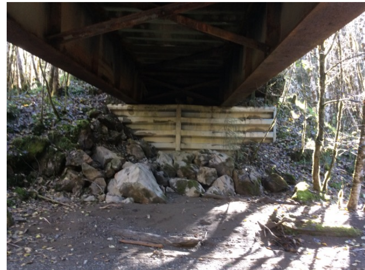
Left Bank Abutment when facing downstream
