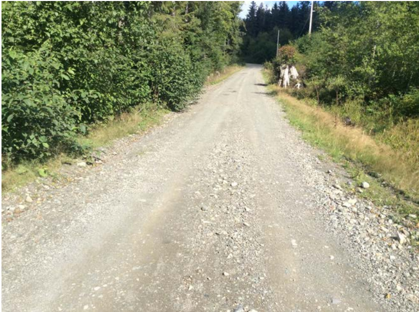
Centre of bridge to river left approach
