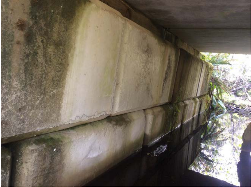
Left Bank Abutment when facing downstream
