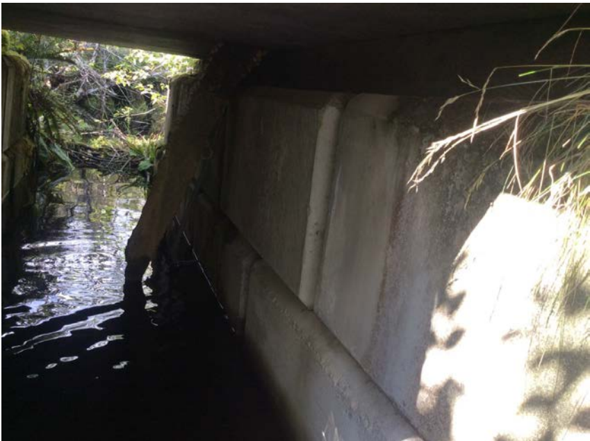
Right Bank Abutment when facing downstream
