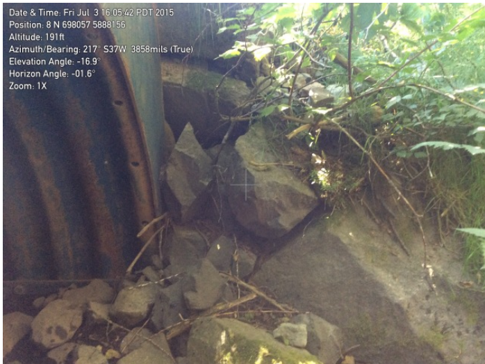
Left Bank Abutment when facing downstream
