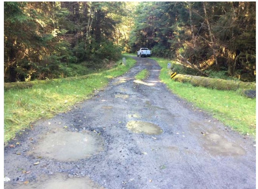
River right approach to Bridge
