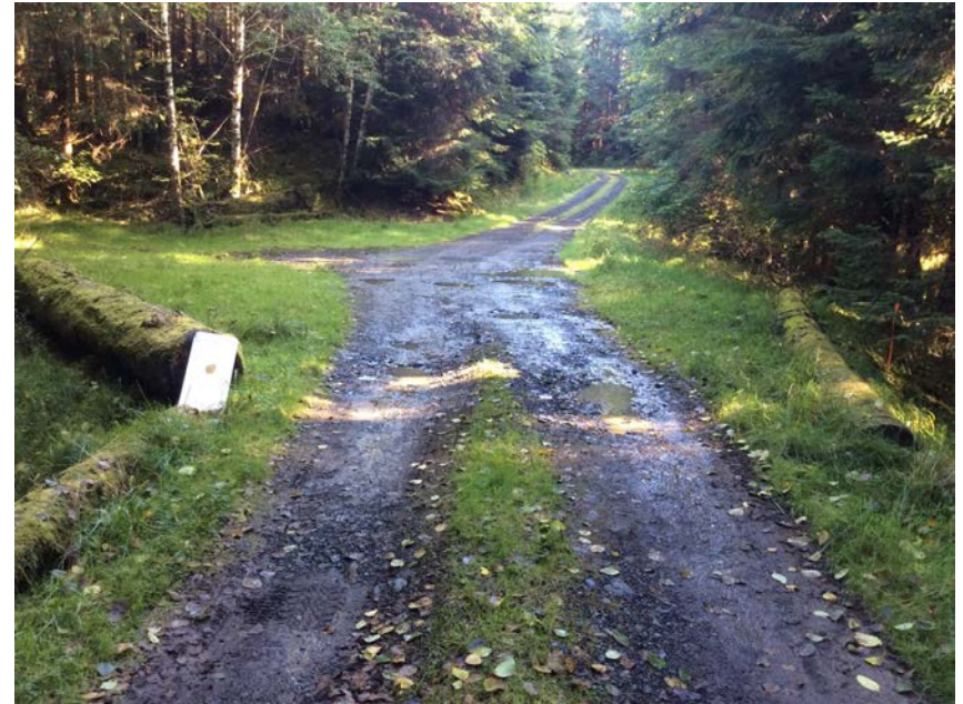
Centre of bridge to river left approach
