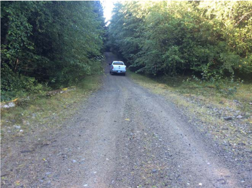
Centre of bridge to river right approach
