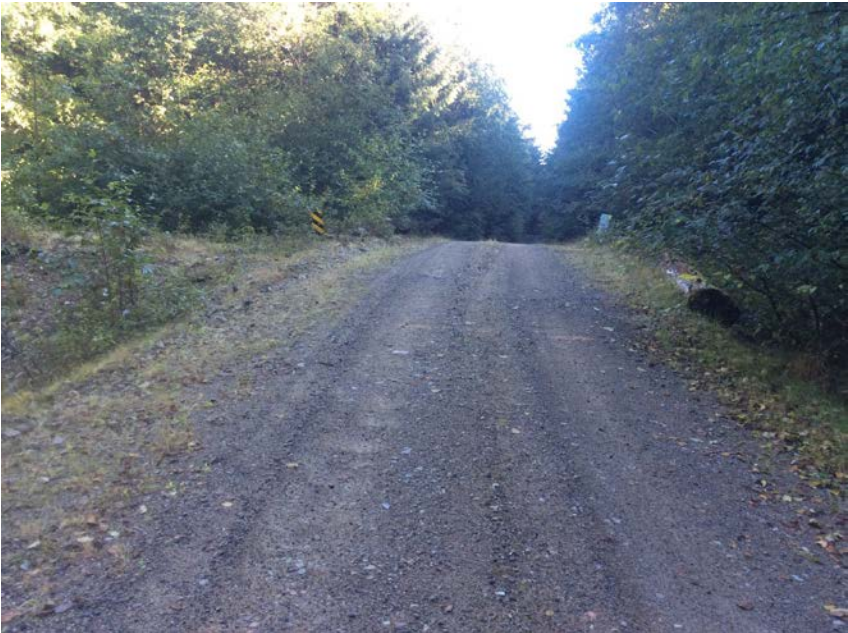
River right approach to Bridge
