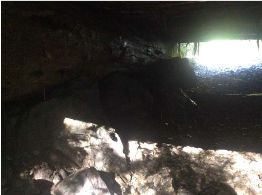
Right Bank Abutment when facing downstream
