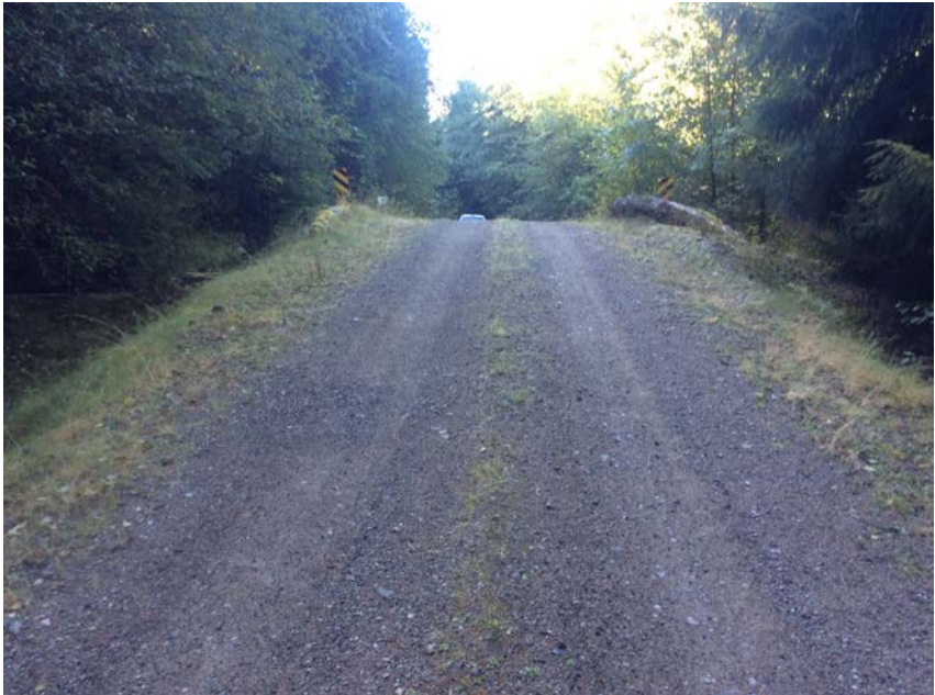
River left approach to Bridge
