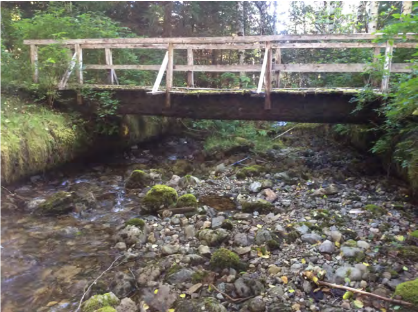
Upstream Profile of bridge 2
