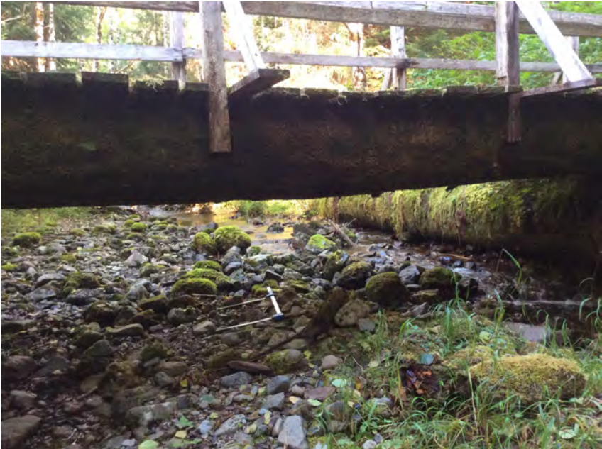
Downstream Profile of bridge 2
