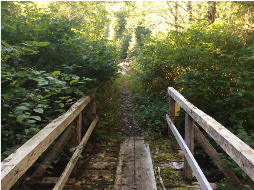
Centre of bridge to river right approach 2
