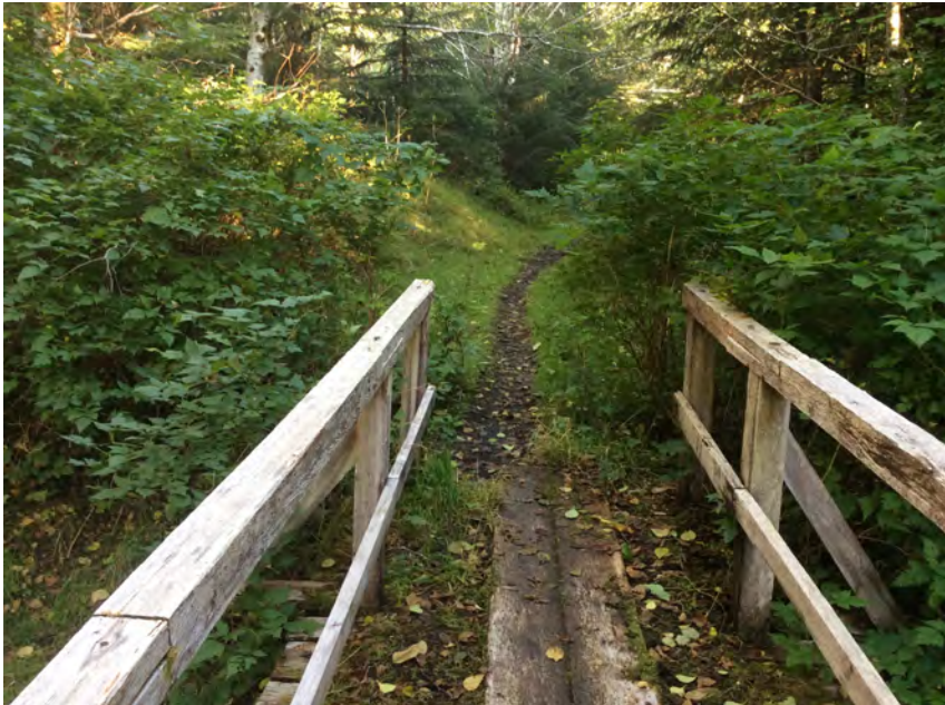
Centre of bridge to river left approach 2
