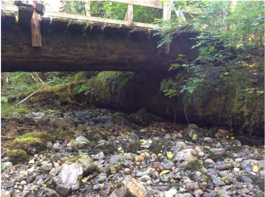
Right Bank Bridge 2 Abutment when facing downstream
