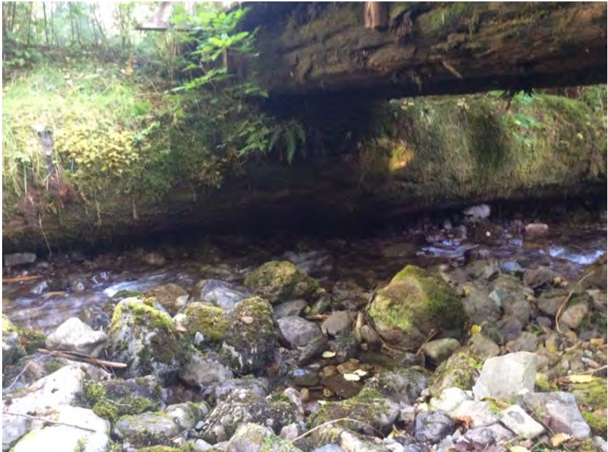
Left Bank Bridge 2 Abutment when facing downstream
