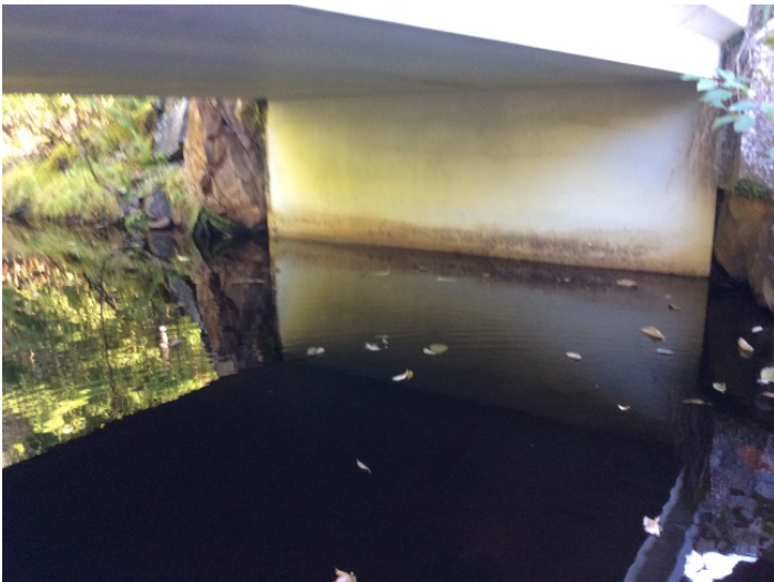
Left Bank Abutment when facing downstream
