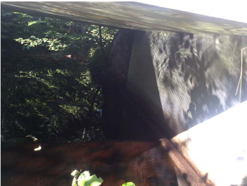
Right Bank Abutment when facing downstream
