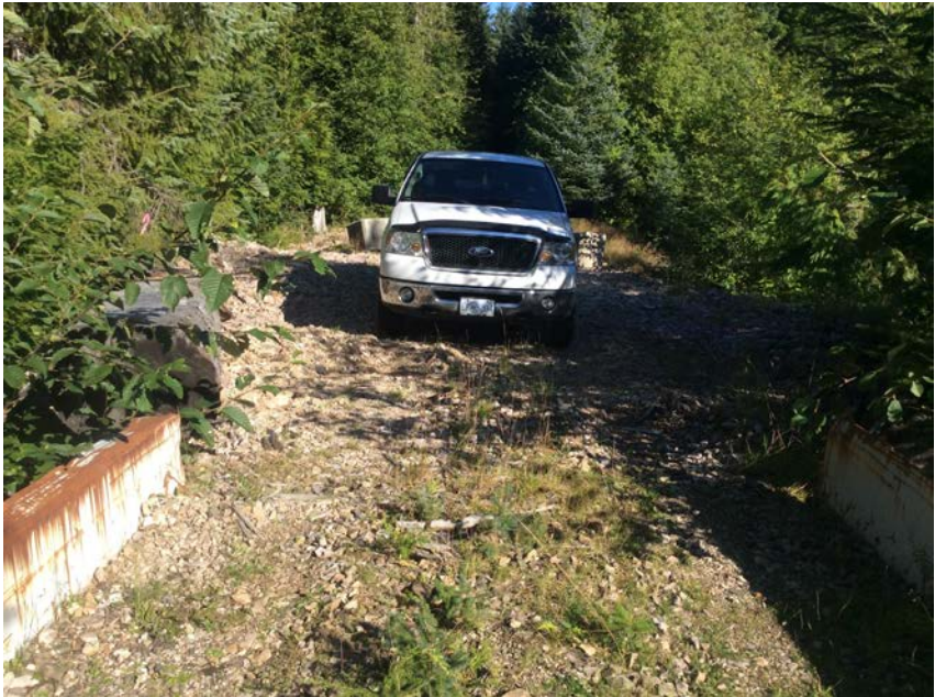
Centre of bridge to river right approach
