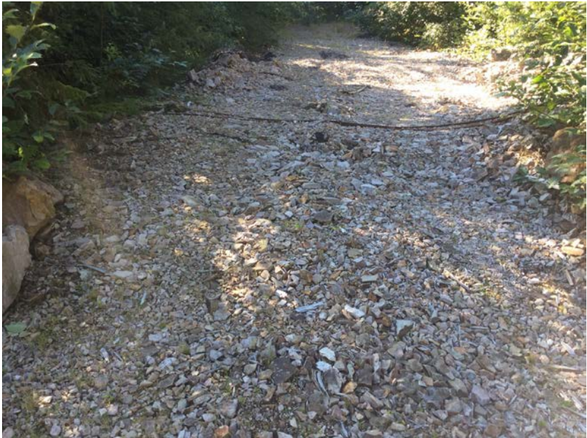
Centre of bridge to river left approach
