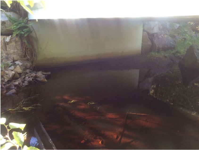
Left Bank Abutment when facing downstream
