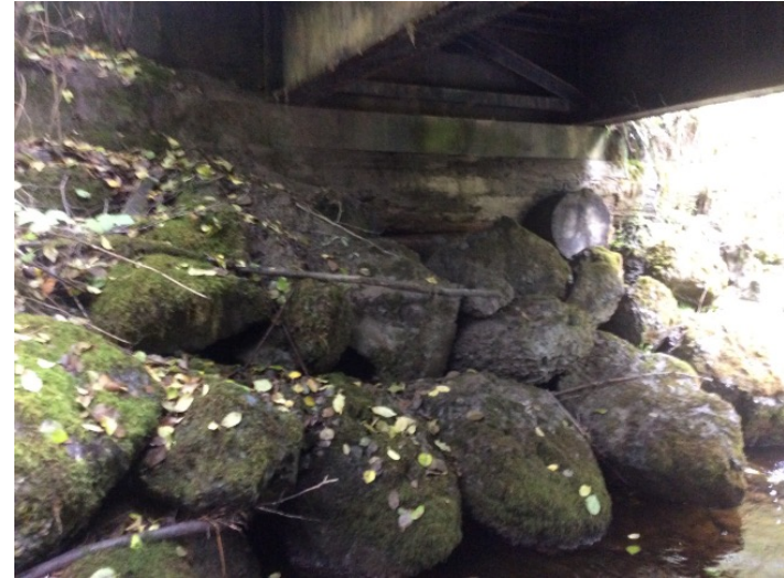
Left Bank Abutment when facing downstream
