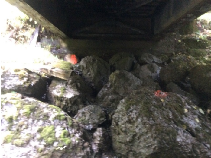
Right Bank Abutment when facing downstream
