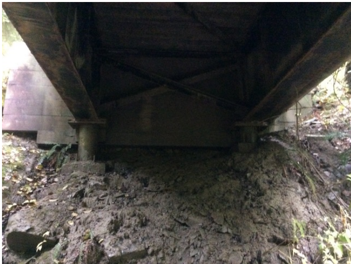
Left Bank Abutment when facing downstream
