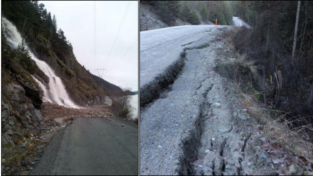
Figure 9. Rocks and water fall onto the in-SHUCK-ch FSR (left), and narrowed road width due to fill slope failures (right). (Source: FSR overview presented at in-SHUCK-ch PIEVC workshop, Squamish, B.C.).
