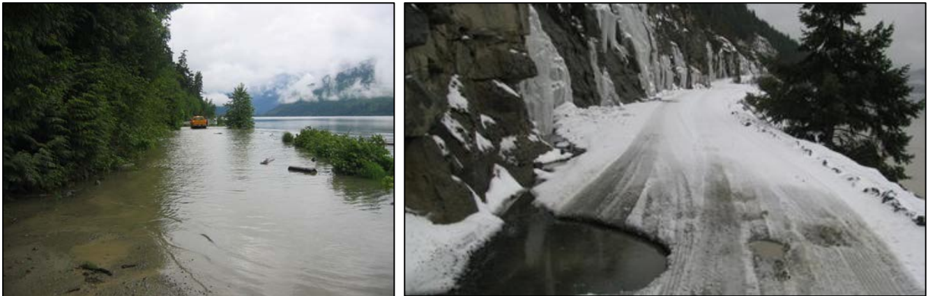
Figure 6. Flooding of the FSR at the south end of the Lillooet Lake (left), and ice flows down rock cuts and onto the FSR cause dangerous driving conditions (right). (Source: FSR overview presented at in-SHUCK-ch PIEVC workshop, Squamish, B.C.).
