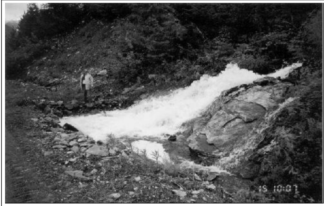
Figure 4. Large seasonal stream flow, relative to 600 mm culvert. Peak flows escaped down the ditch towards top of photo, causing the landslide shown in Figure 5.
