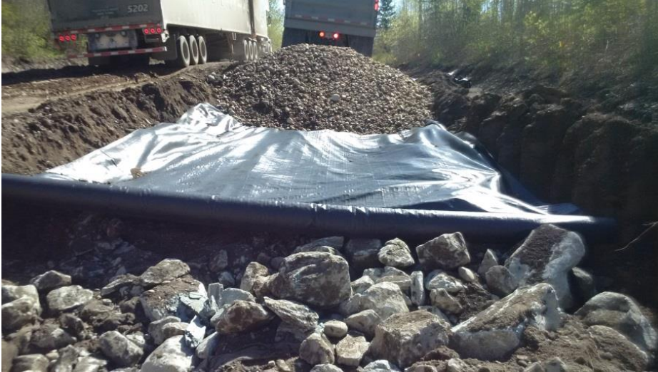
Figure 6. Reconstruction on the KM 11 hill of the Willow FSR with a free-draining subbase (photo courtesy of Carrier Lumber).
