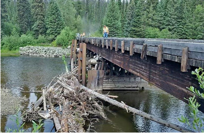
Figure 4. Minor logjam in July 2018 rests against guard piles of Willow River bridge (KM 51.4).
