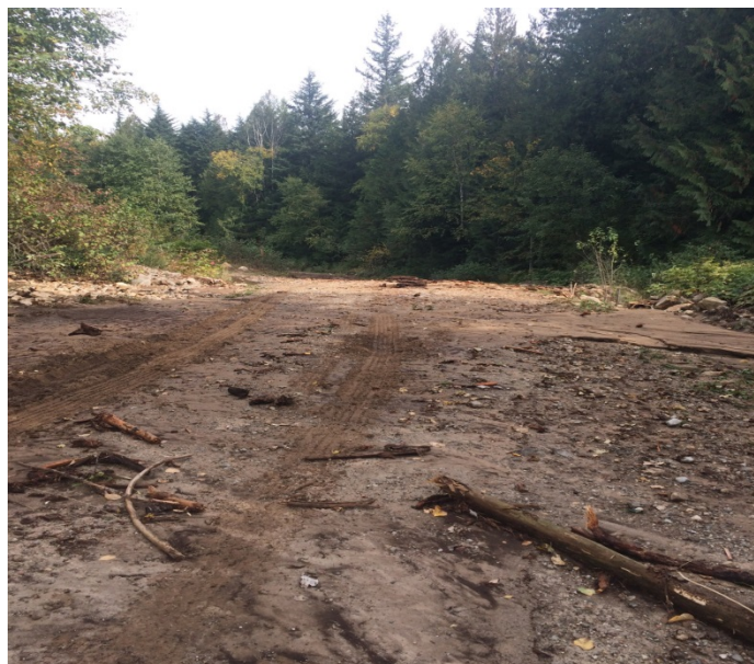
Figure 4. The road surface from KM 17.3 to 21 required repair following storm damage in September 2015. Photo courtesy of Daryll Cairns.
