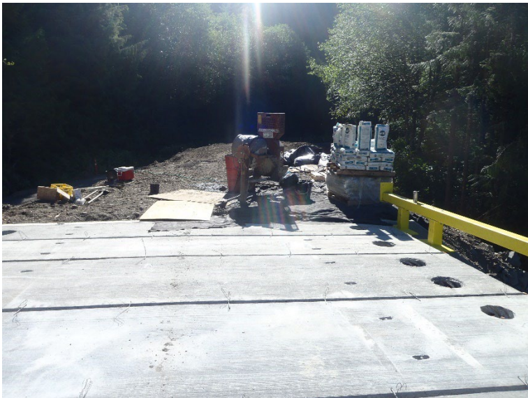
Figure 7: Batch of CIP mixture in a mixer, to be used for shear stud blockouts for deck panel to girder connections on a new steel girder composite concrete deck bridge.
