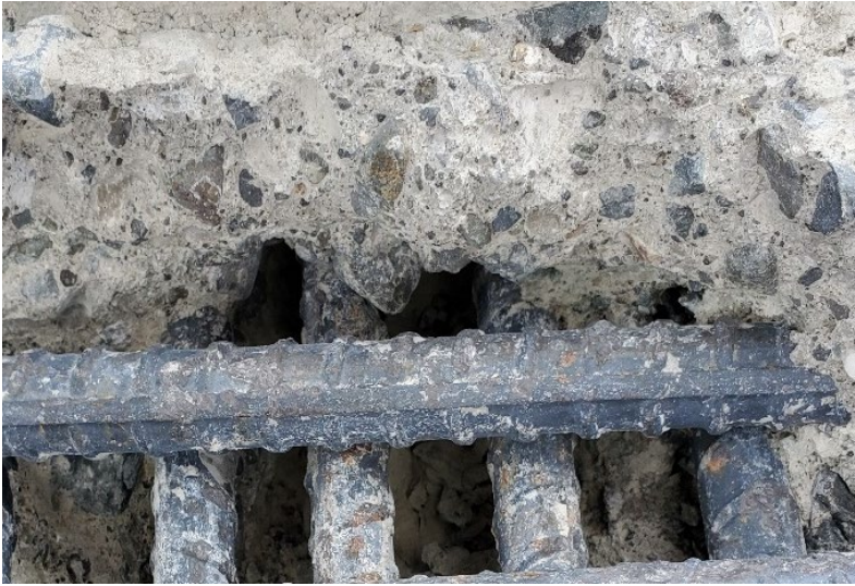
Figure 4: An example depicting a typical surface roughness profile of CSP 10. Coarse aggregate surfaces are well exposed and free of loose concrete, sand, dust and debris.
