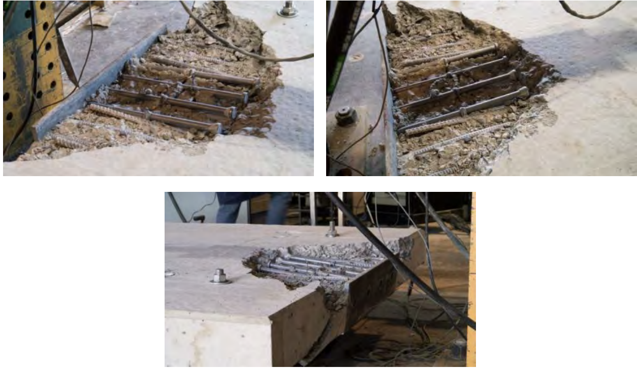
Figure 41: Images from G-1-1, failure inspection after top concrete removal
