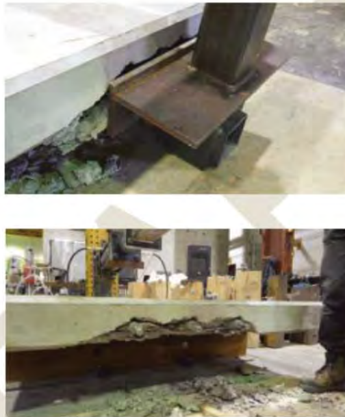
Figure 2 Typical Observed Failure of the Modified HSS Guide Retrofit Rail
