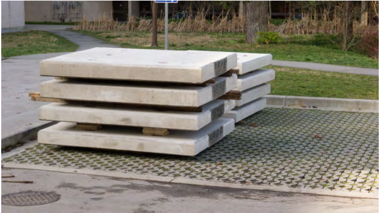
Figure 3: Panels Stored Outside
