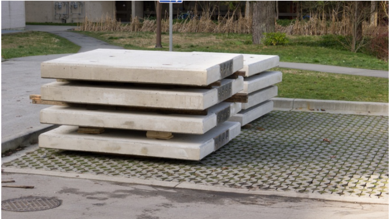
Figure 3: Panels Stored Outside
