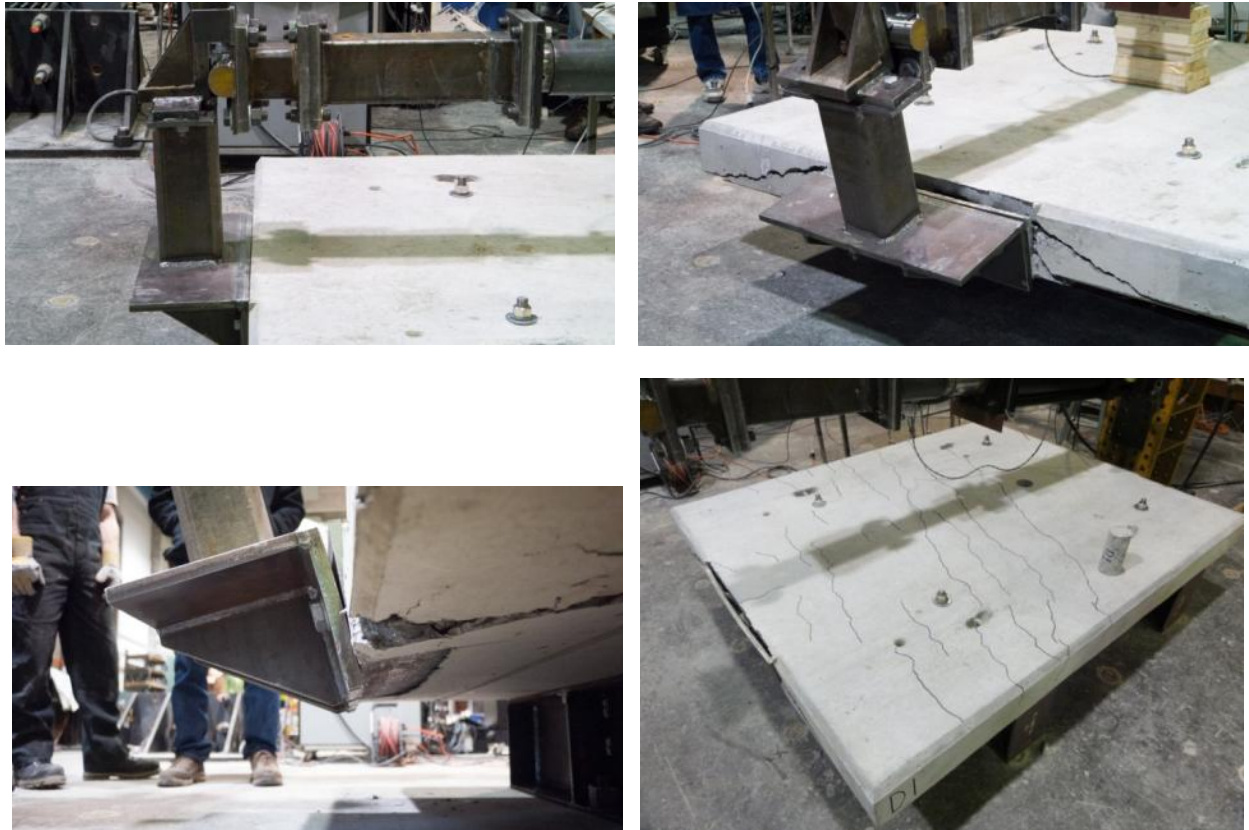
Figure 22: Concrete panel attachment detail failing
