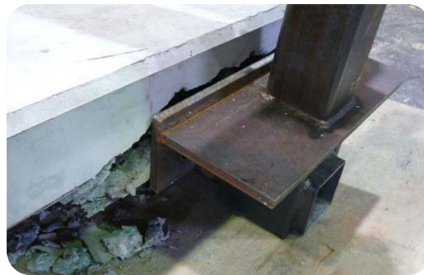
Side Mounted Steel Bracket with Knee-Brace Modification
