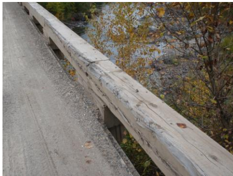
(A) Timber Curb
