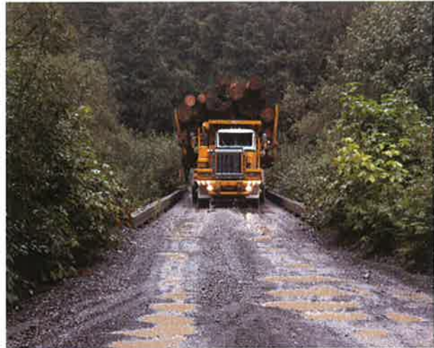
Off-highway logging truck crossing a 4.8 m wide bridge
