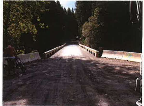
Approach barriers on a heavily trafficked bridge with significant public usage
