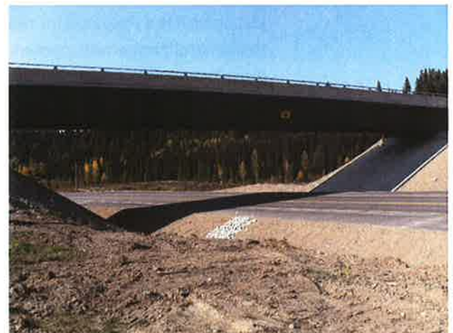
Bobtail FSR highway overpass
