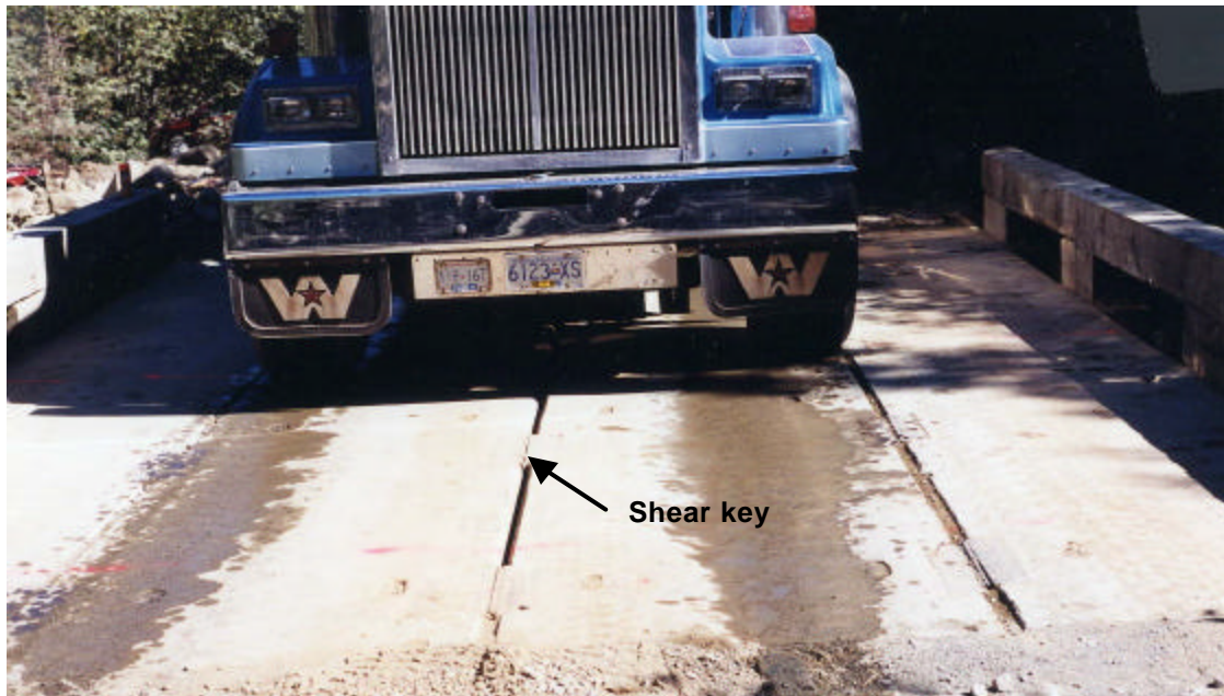
Figure 1 A typical shear-connected concrete plank bridge in British Columbia
