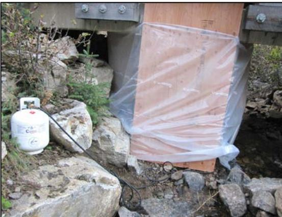
*Figure 9: Makeshift tent used with a Tiger Torch to provide heat in cold temperatures to improve grout curing conditions for the repair site. This method is known as 'hoarding'.*
