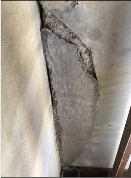
*Figure 8: Formwork on underside of deck panel removed showing grout patch inadequately tamped along the edge of the formwork; see Figure 7 for additional repair.*
