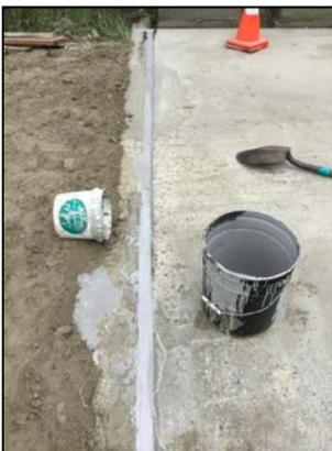
*Figure 12: Paraseal sealant placed at gap between ballast wall and concrete deck subsequent to concrete repair works.*
