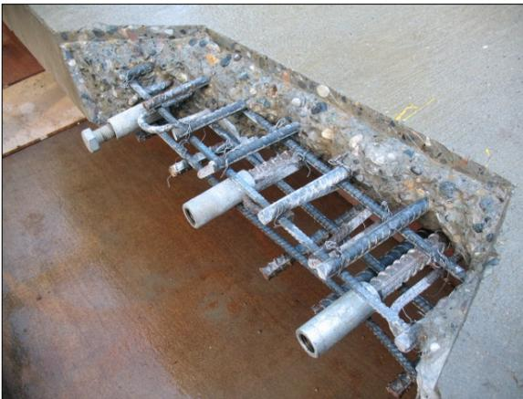
*Figure 5: Ready for formwork. Exposed rebar after damaged concrete removal; note saw cut square edges.*
