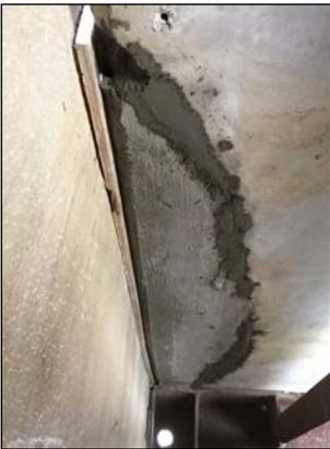
*Figure 11: Additional grout patch being placed into bottom of a deck panel, adjacent to a ballast wall, to fill voids from initial unconsolidated repair work to obtain original deck dimensions*
