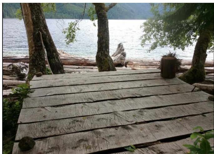
Figure 10: Tenting platform at Blackie's Beach
