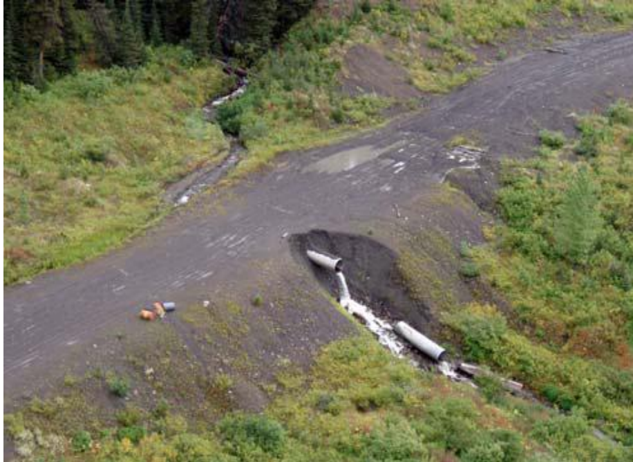
Photo 13. Typical culvert along the rail grade in the upper Skeena area
