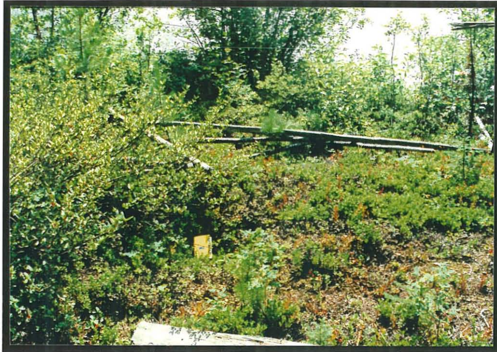
Plate 3: Area 2 – Fallen structure(s) and associated (?) cache pit (yellow note book in cache).
