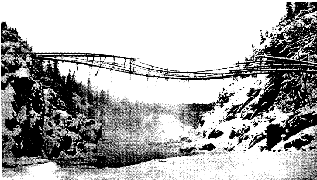
Plate 5. First Bridge at Hagwilget (1872). (BC Archives)
