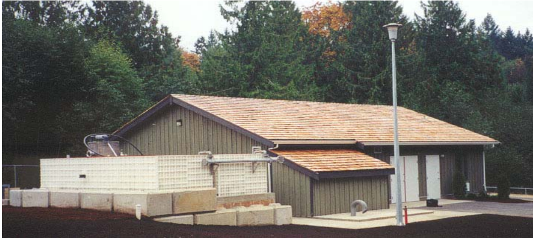
USBF Bioreactor modules (2) and Process building
