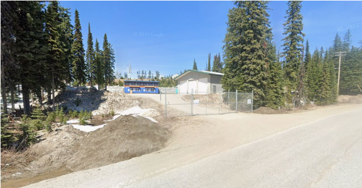
Photo 5: Transfer station at located on Big White Road operated by the RDKB
