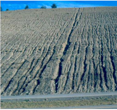
Example of rill and gully erosion.
