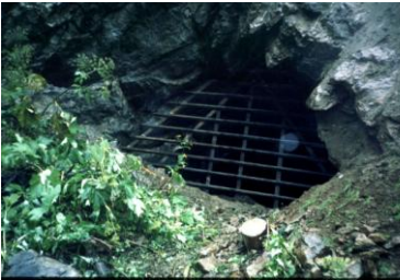
Mine opening closed with rail salvage. This allows passage for bats, permitting their colonization of old workings.
