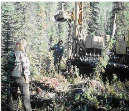
Nodwell mounted auger drill.
