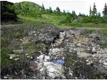
Small trench in alpine site excavated by heliportable excavator.
