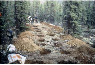
Trenching using explosives.
