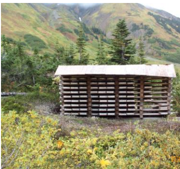
Core storage built for long-term use and able to withstand snow loads.
