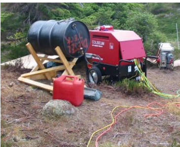
Camp generator and fuel. Note several items for improvement: the horizontal fuel drum, small drip tray, and lack of blanket material to absorb any fuel leaks
