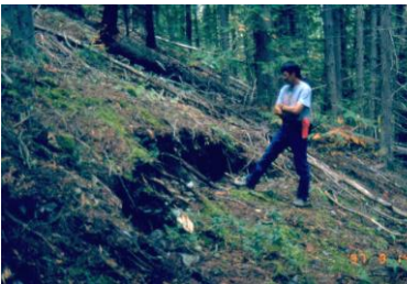
Tension cracks on steep slope.
