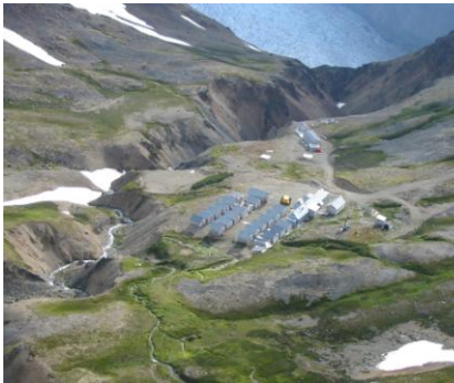
Camp for a large MX project. Camp access was via air transport and given the elevation, care was taken to construct the camp to withstand snow loading.
