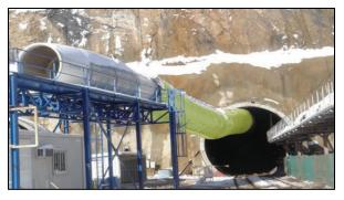
Positive pressure ventilation uses a fan to create a high-pressure zone. In underground operations, this is done by placing a fan at the entrance of a tunnel, facing inwards. The high-pressure air in front of the fan will flow to the lower pressure areas further from the fan. The scooping action of the fan blades prevents the air from flowing back through the fan.
