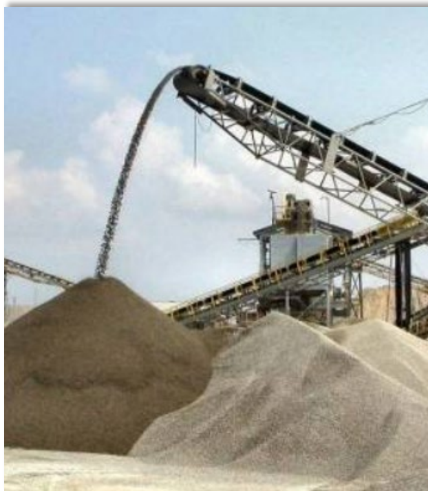
FIGURE 15: STOCKPILE BENEATH HEAD PULLEY
