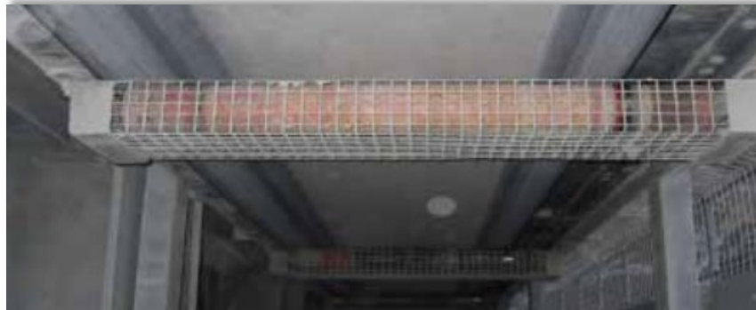
FIGURE 3: GUARD PROTECTING A RETURN IDLER
