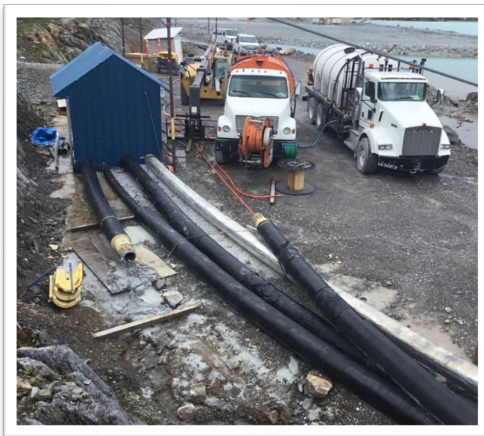
FIGURE 1. Line blocking work area where incident occurred.
