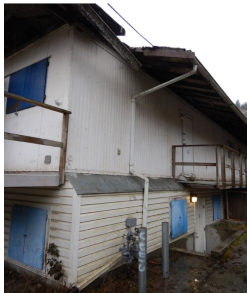
FIGURE 1. Roofing works, Incident Scene
