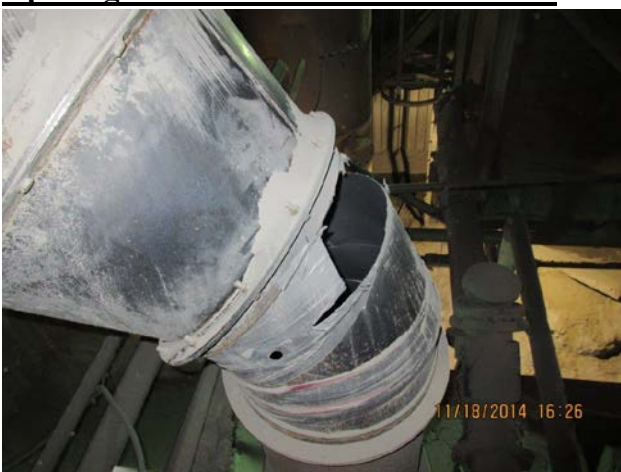
Opening in main duct SE side of crusher
