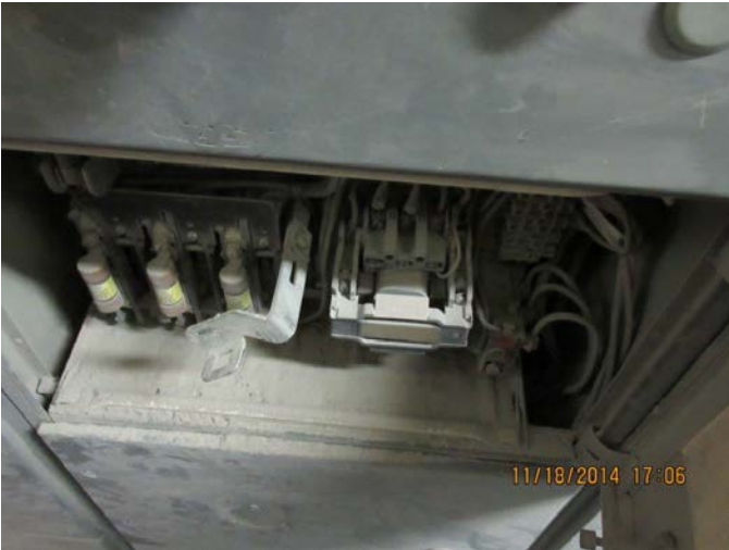
Dust contaminated switch lower MCC room N end of crusher by primary crusher
