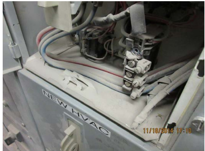
Dust contaminated switch lower MCC room
