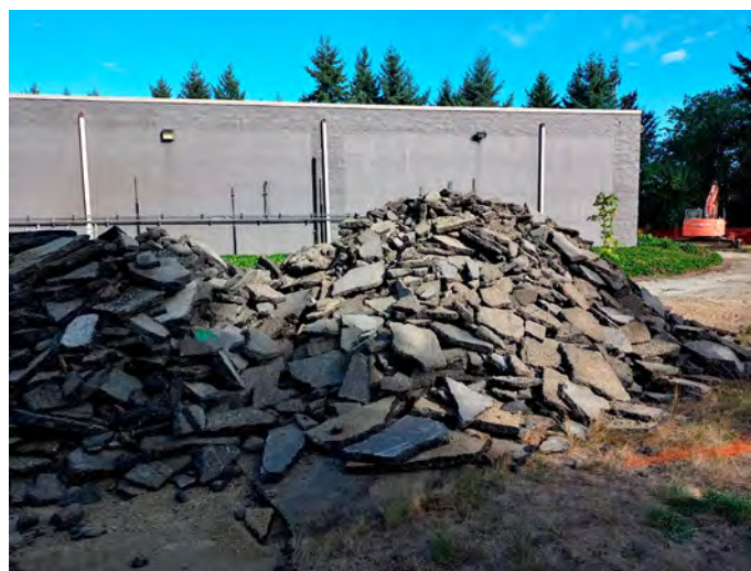
Figure 2. Breaking ground, September 19, 2023.
