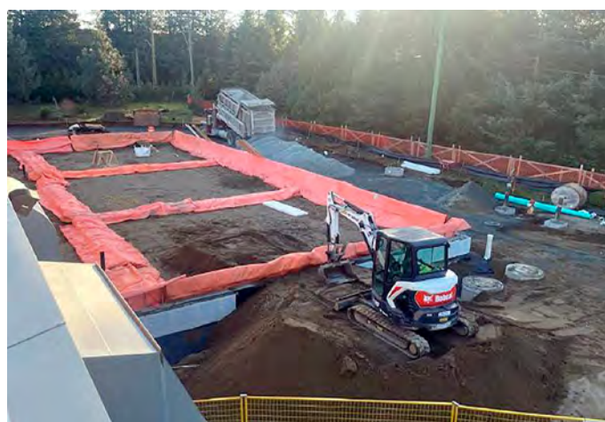
Figure 3. Initial interior and exterior wall construction, Fall 2023.
