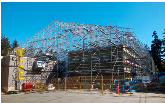
Figure 5. Final new building height inside the scaffolding, as weatherproofing began.
