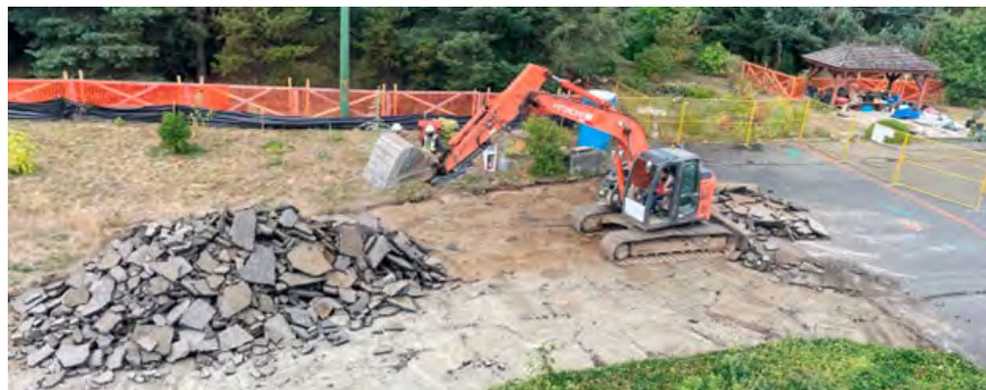
Top: Artist's rendering of the BC Tree Seed Centre freezer and cooler expansion project (new additional space underlined in red). Bottom: Breaking ground, September 18, 2023.
