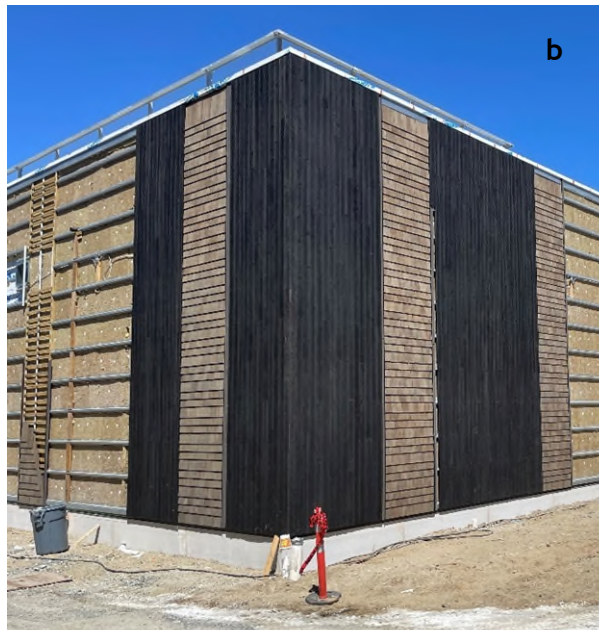
Figure 1: a & b. The new and older exterior of the brick framework for the freezers and coolers was covered in a vapor barrier, rock wool insulation and then covered with wood cladding.
