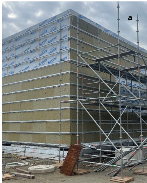
Figure 1: a & b. The new and older exterior of the brick framework for the freezers and coolers was covered in a vapor barrier, rock wool insulation and then covered with wood cladding.
