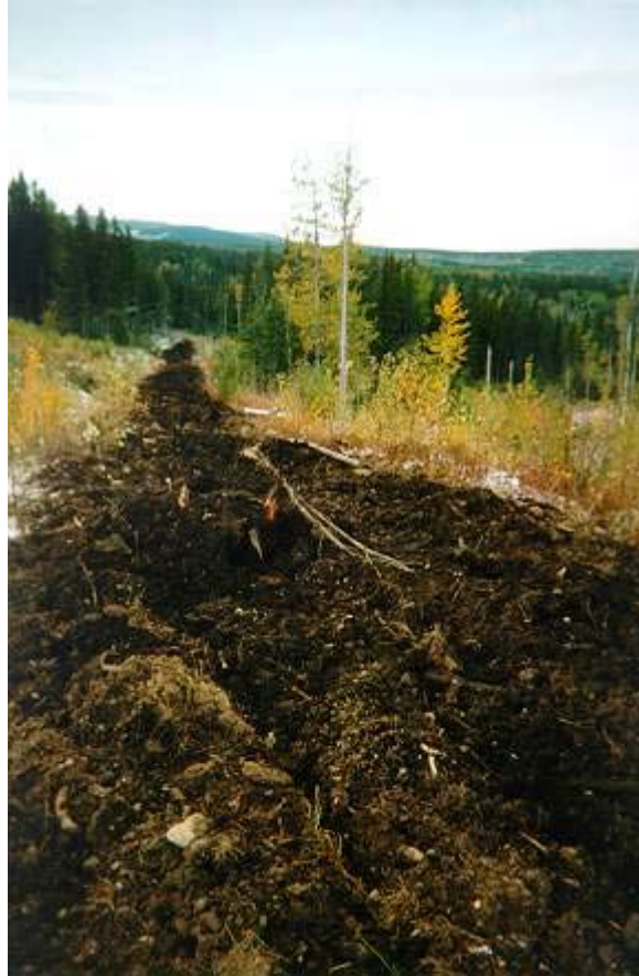
Photo 3: Temporary roads are rehabilitated to minimize reductions from the landbase.
