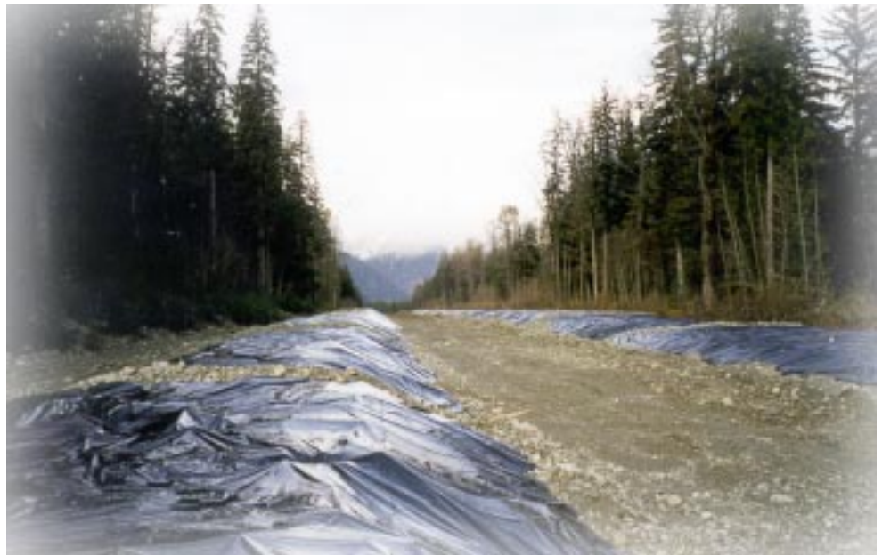
There are two biocells over 800 metres long running on both sides of the Kimsquit airstrip photo: Corby Lamb
