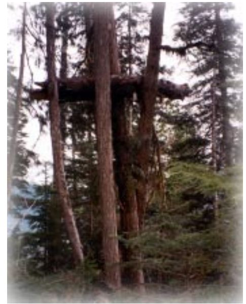
"Widowmaker" danger tree
