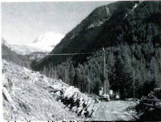
Photo: Schiller Contracting's Goft Madill tower in CP 143-2 Downie Creek.
