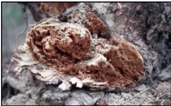
End view of decay caused by O. tomentosa (Photo credit R. Reich).
