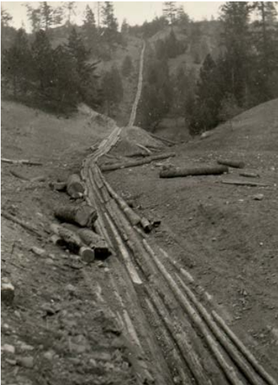
b. log chute in ponderosa pine forest near Monte Lake; logged area with residuals in background
