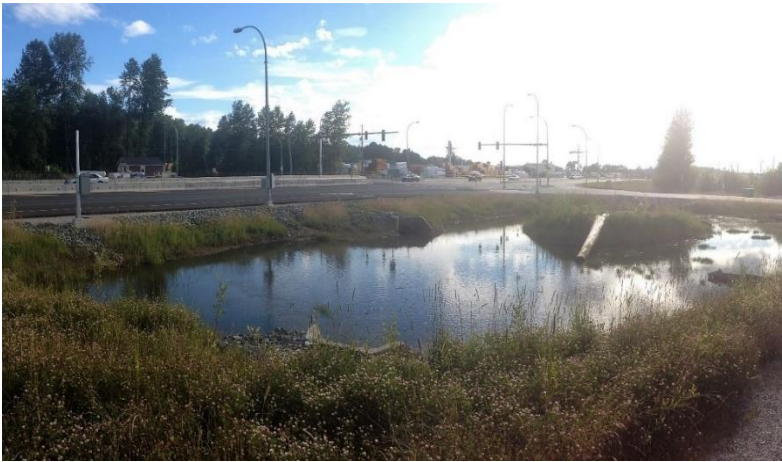
Figure 16. Highway directly adjacent to a wetland, which leads to high levels of noise pollution, runoff into the wetland and has no accommodations for wildlife access.
