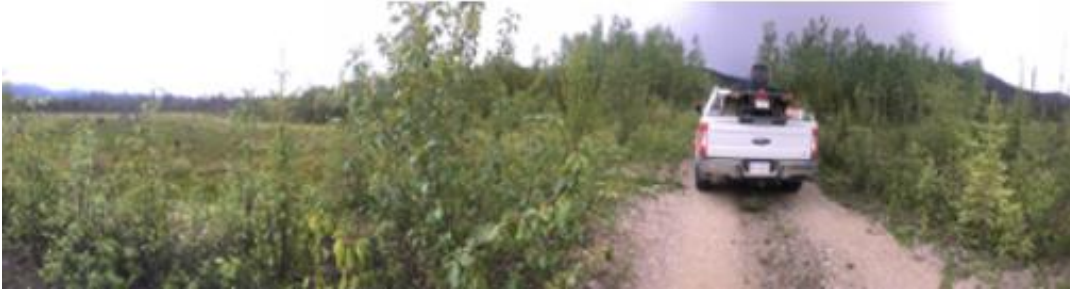
Figure 15. Forest Service Road crossing through a wetland. Insufficient culverts led to pooling of water upstream (left), and more vigorous growth and shrinking of wetland on right hand side.
