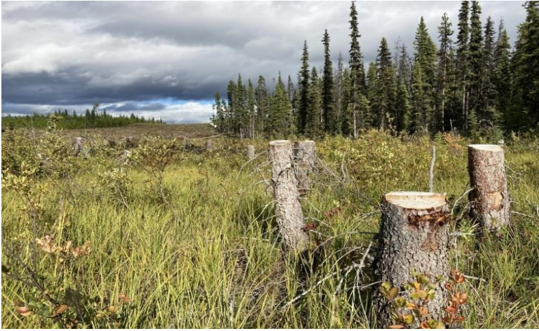
Figure 20. Forested wetland cleared for pipeline ROW.
