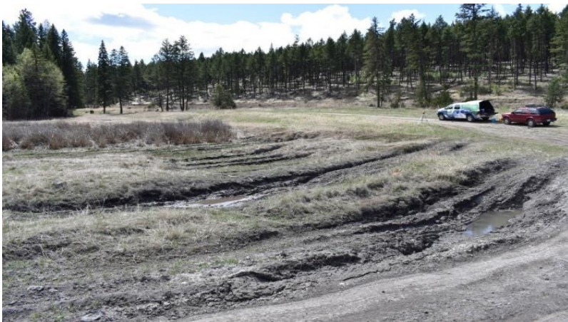
Figure 19. Rutting and compaction by off-road ATV and 4X4 users.
