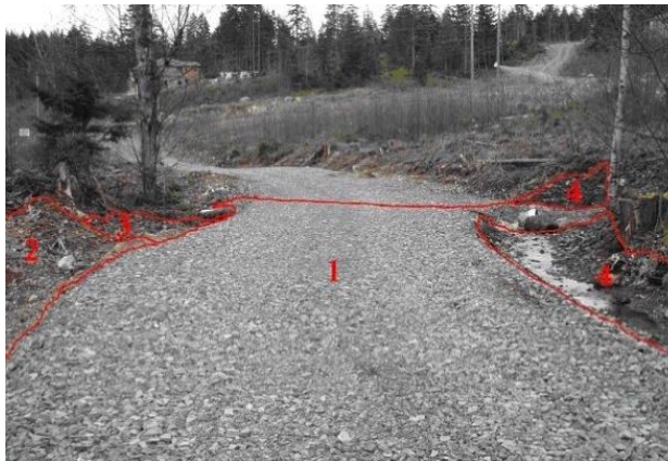
Photo 1. Downstream view of a culvert crossing on an S6 stream. The stream flows down the right side ditch, then across the road from right to left. The red lines and numbers delineate areas that are similar with respect to the amount of bare erodible ground exposed and the degree of hydrological connectivity to the stream.
